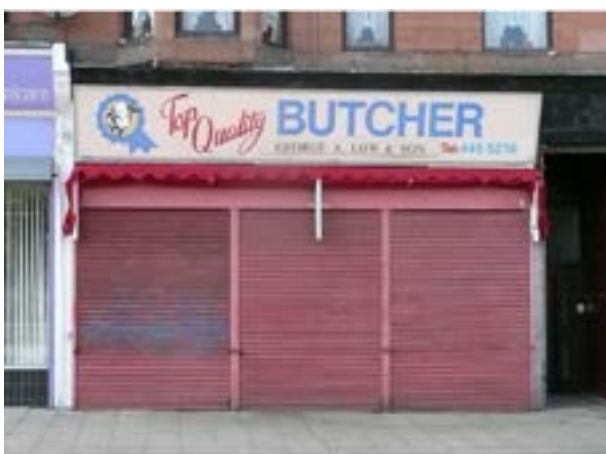
The solid roller shutters create a 'dead' shopfront when they are closed.
