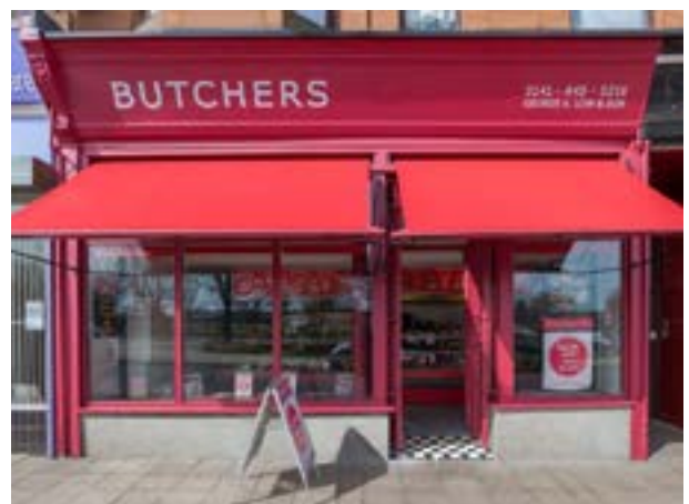
Toughened, laminated security glass has been used instead of shutters.
