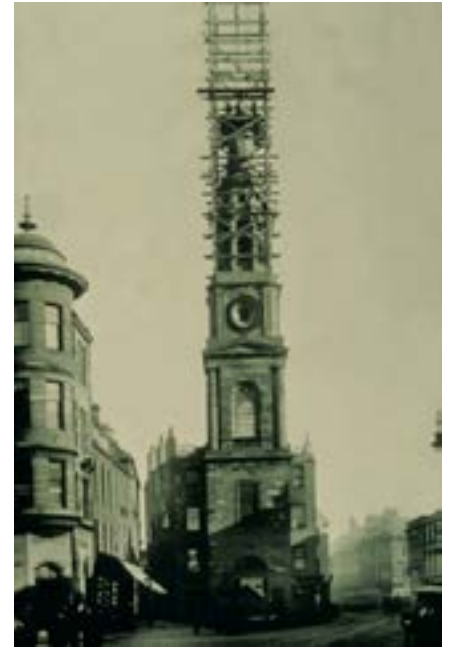
Falkirk Steeple being rebuilt after it was hit by lightning, 1927 (P14967)
