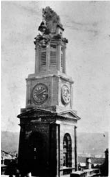
The damage to the top of Falkirk Steeple after it was struck by lightning in 1927 (P02840)
