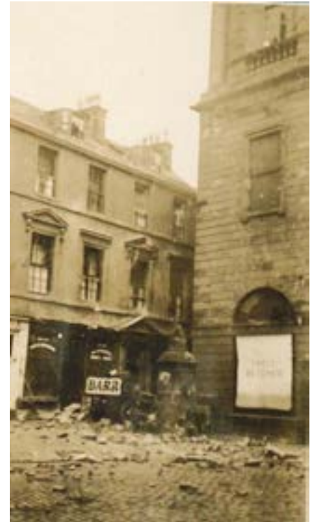
Fallen masonry and Barr wagon in High Street after Falkirk Steeple struck by lightning.
