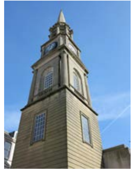
2013 View of Falkirk Steeple
